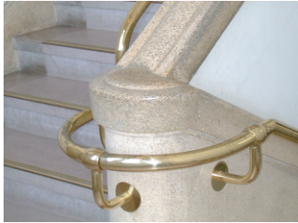
Handrail with exposed aggregate by honed stone finish.
