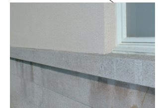
Exterior wall with exposed aggregate finish by brushing (upper part) and by washing (lower part). The lower grey wall was built using an exposed aggregate finish by washing, i.e. built using mortar mixed with stones and then lightly watered to wash off the mortar on the surface before the cement hardened for the stones to surface. The upper wall was built using an exposed aggregate finish by brushing, i.e. brushing off the surface before the mortar dries.
