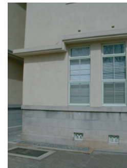
Vertically long windows, a pre-war building feature, and concavo-convex structure on the wall.
