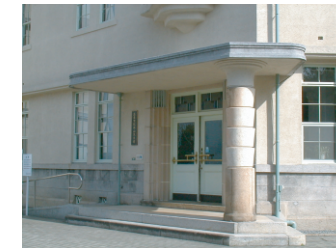
Pillar with stacked inverted cones with a honed stone finish, which is hardly found today. Unconventional thin eaves supported by a single pillar challenged the mainstream design of the time.
