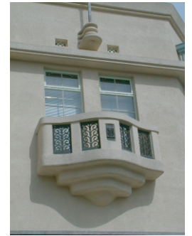
The simple-design modern window sill of the balcony and the characteristic design flag pole stand above.
