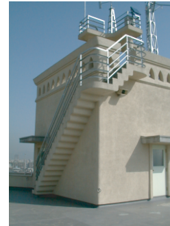
Cantilever staircase leading to the roof of the observatory.
